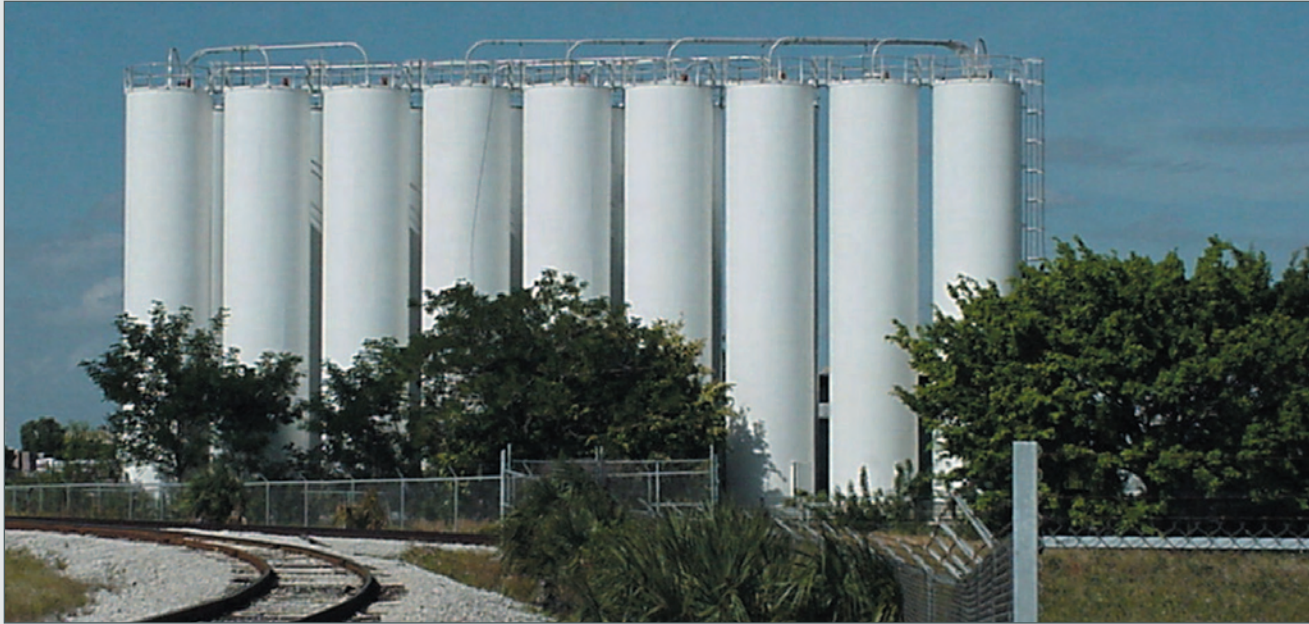
Silo farm for large plastic processor.
