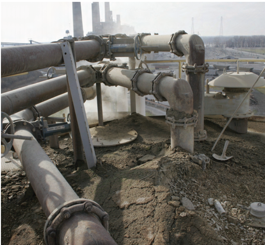
Roof of silo at fly-ash processing plant
