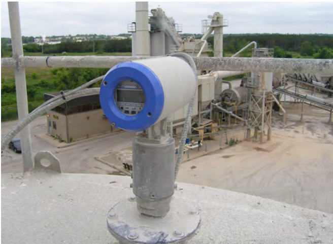
Figure 1. A Flexar ® guided wave radar level sensor being used in a concrete batch plant
