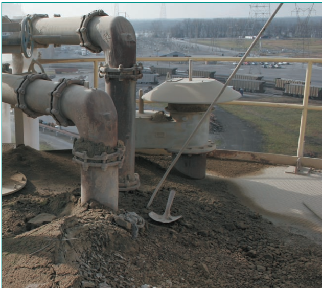
Figure 1. Roof of flyash silo.
