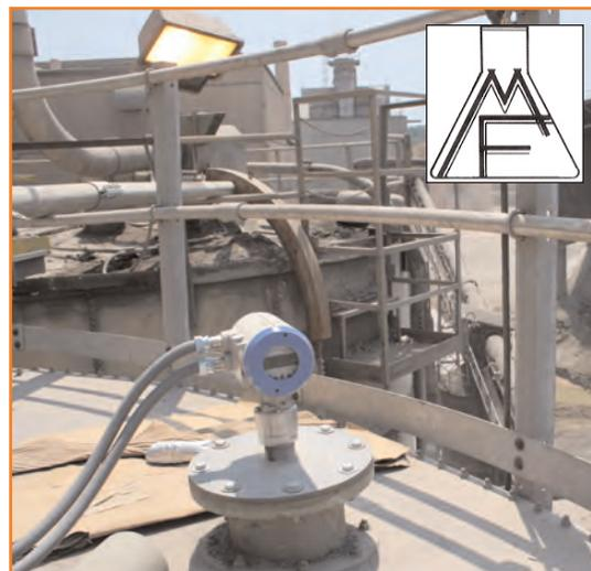
it wasn't a surprise when Quenton got the opportunity to meet their needs on the flyash silo. Flyash is a powder and the internal silo atmosphere during filling is extremely dusty, but Schott knew he had a solution for his customer. After quickly consulting with Monitor Technologies, the Flexar™ guided wave radar continuous level sensor was recommended and quoted.
