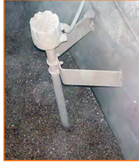
Example of a rotary paddle switch with an extension and guard
