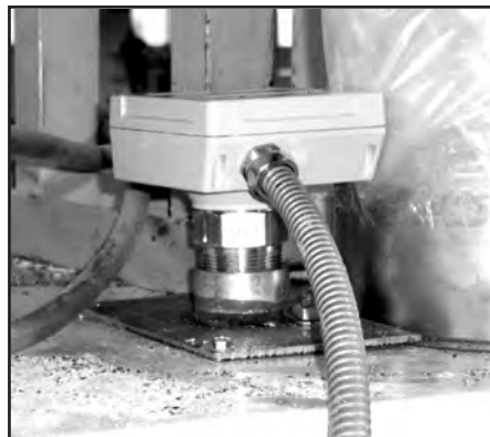
This PZP is being used as a high-level alarm in a plastics application. The PZP was ideal for this application because of its reliability with light weight materials.
